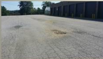
FBE, CHS and HAE Overlay/re-pave asphalt parking lots and drives
