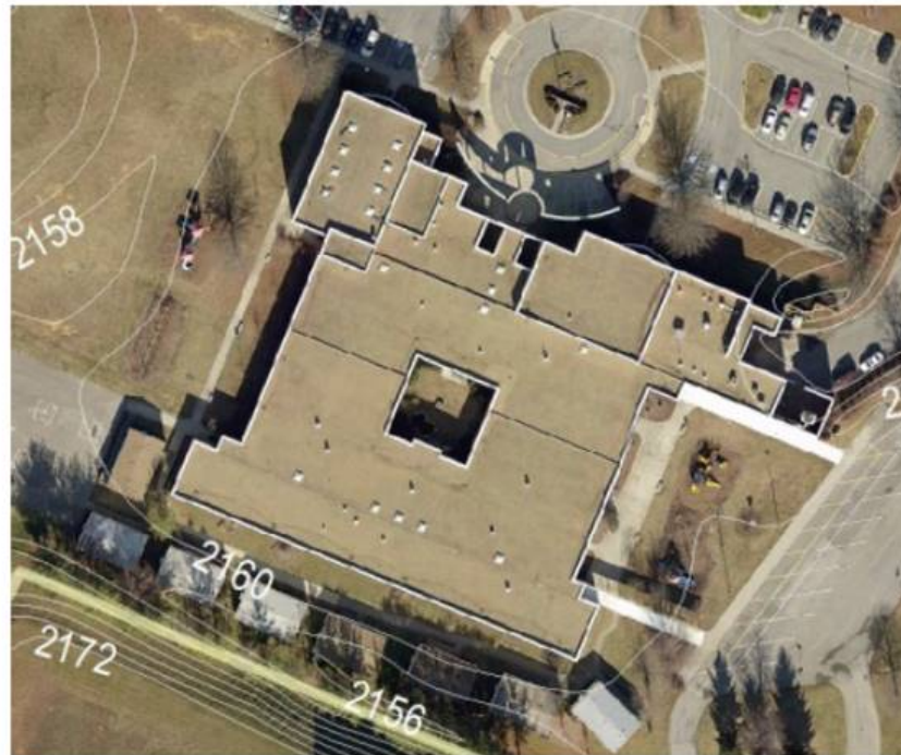
Falling Branch Elementary Main Roofs
