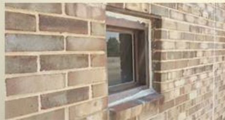
CHS Replace Library Windows CT
