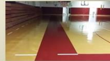
SMS Replace gym floor and bleachers
