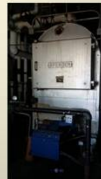
CPS Install new boiler - CT
