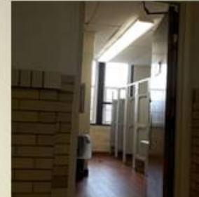
SMS and FBE Replace bathroom partitions
