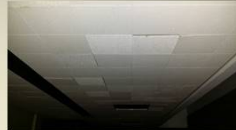
CHS, SMS Replace ceiling tile
