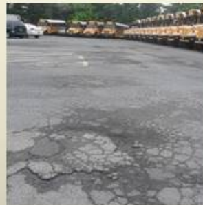
Cambria, Technology Pave/overlay asphalt parking lots
